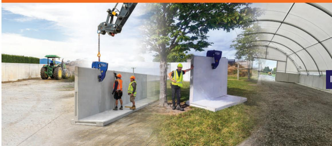
CONCRETE SI-LUTION has mastered the construction of superior concrete walls. Initially designed as a solution for silage bunkers, these versatile freestanding walls are internally strengthened and built to the New Zealand Building Code.
